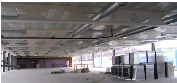
Figure 24a: Angelina® beams in composite floor systems
