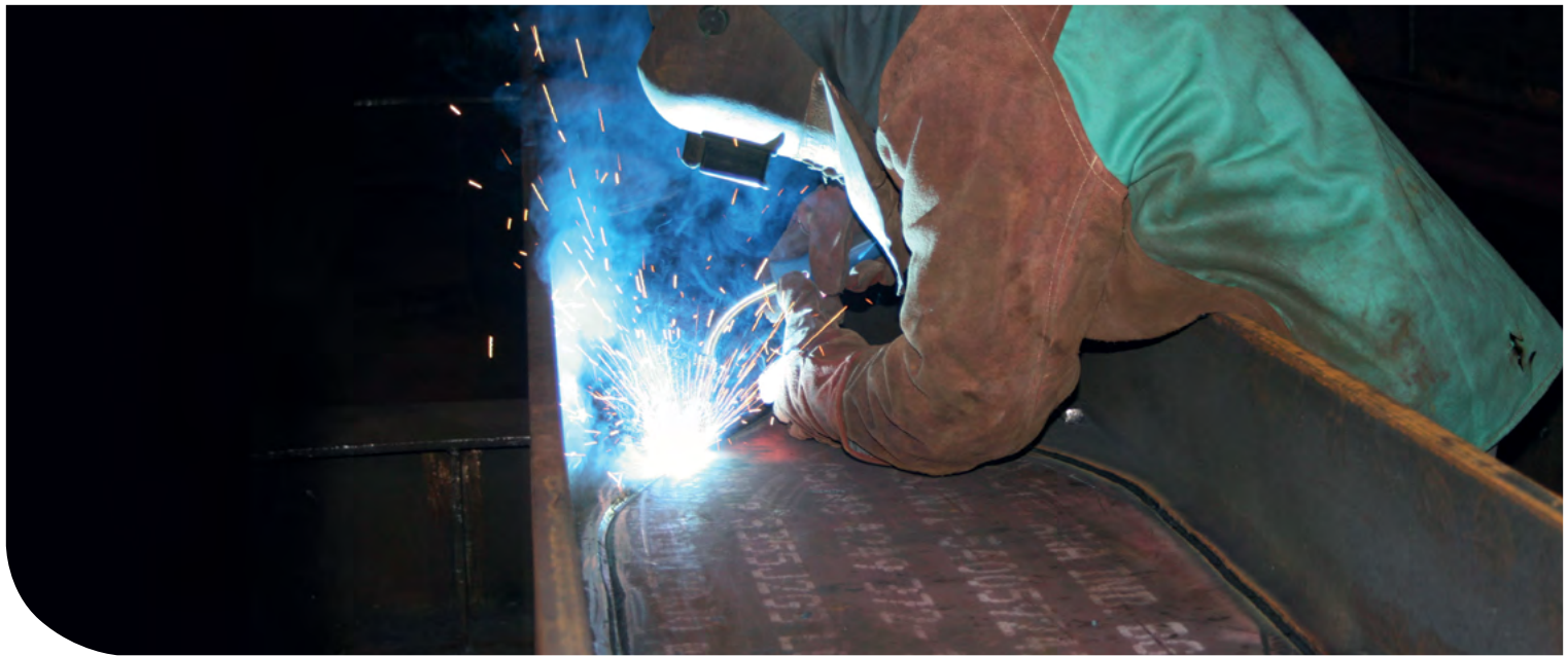
Figure 7: Fabrication of Angelina® beams
